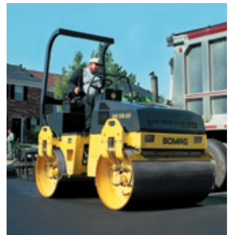
BW138AD in action on an asphalt repair application
